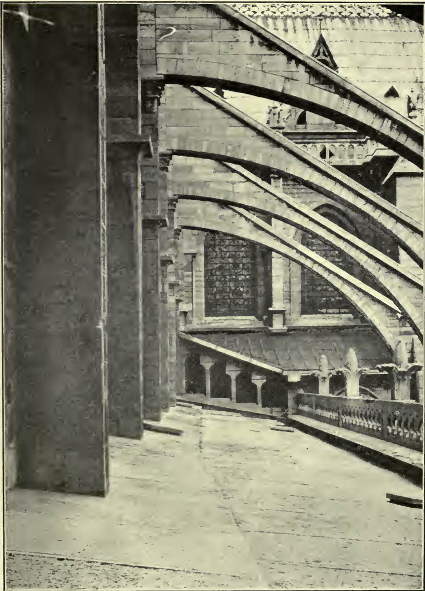
FIG. 10. NOTRE-DAME. ROOF OF THE SOUTH GALLERY, LOOKING EAST.
